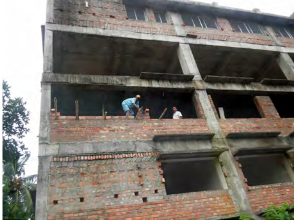
Kolkata Mission Center under construction
