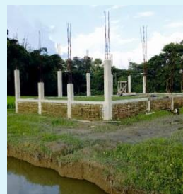
Parul Presbyterian Church Construction
