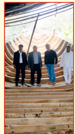
Eternal Life Boat under Construction
